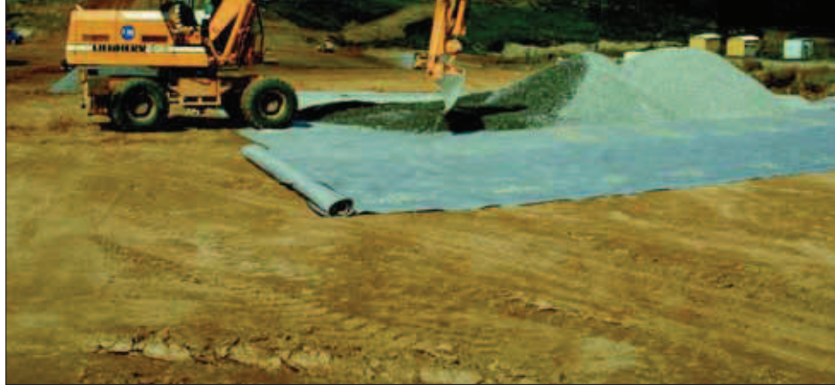
▲ 9 - Anti-contaminant geotextile under a horizontal gravel drain. (text p. 79).
