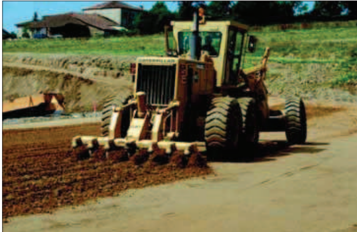
◀ 7 - Scarification after passage of a smooth roller compactor. (text p. 102).
