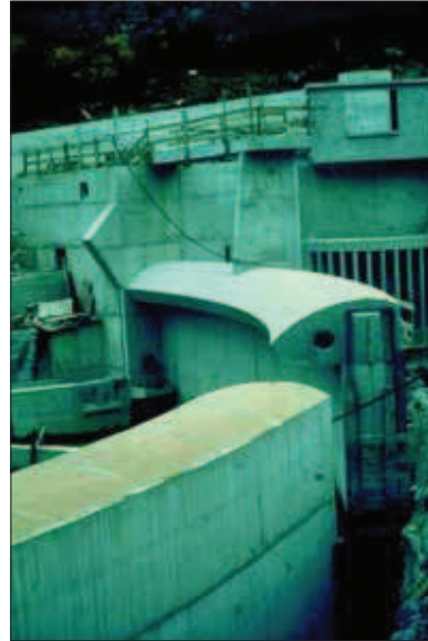
22 - Single curvature arch dam (Chapeauroux water intake). Note the standard crest shape of the overflow portion. (text p.115).
