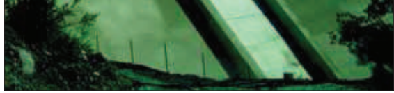
22 - Single curvature arch dam (Chapeauroux water intake). Note the standard crest shape of the overflow portion. (text p.115).
