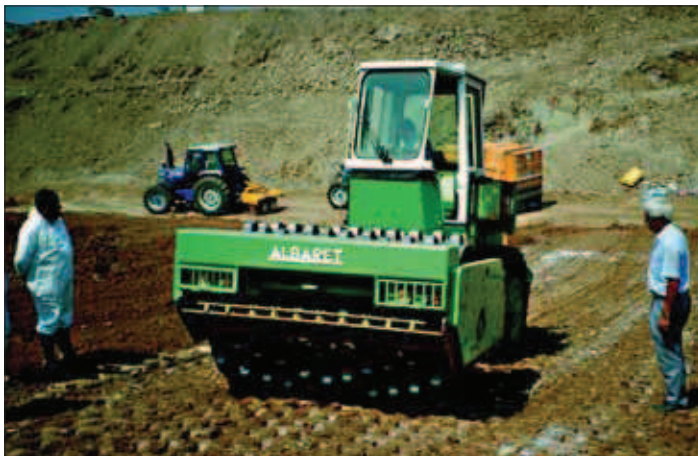
◀ 8 - Compacting with a vibrating tamping roller (scarification as shown above is pointless with this roller). (text 102).
