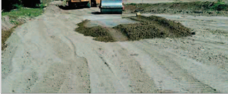
▲ 3 - Test section for a very small dam (at the bottom are the smooth roller compactor and a motor grader conveying earth from the borrow area) (text p. 102).
