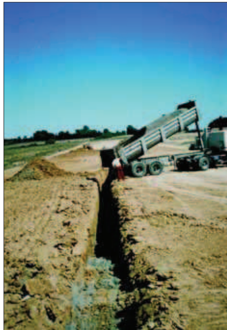
◀ 2 - Vertical drain dug back out of the embankment and filled in with a draining, self-filtering sand (text p. 78).
