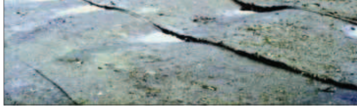
◀ 7 - Scarification after passage of a smooth roller compactor. (text p. 102).
