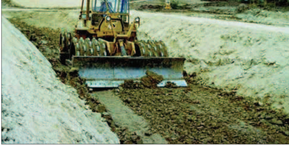
▲ 1 - Compacting clay in the cut-off trench (text p. 71).
