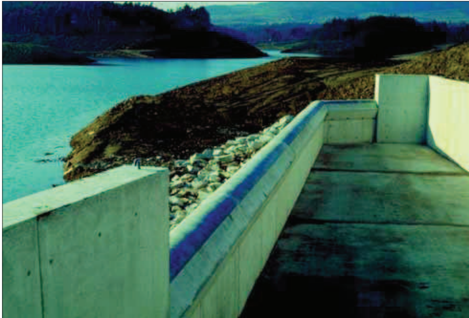
▼ 20 - Overspill part of a side inlet spillway.
