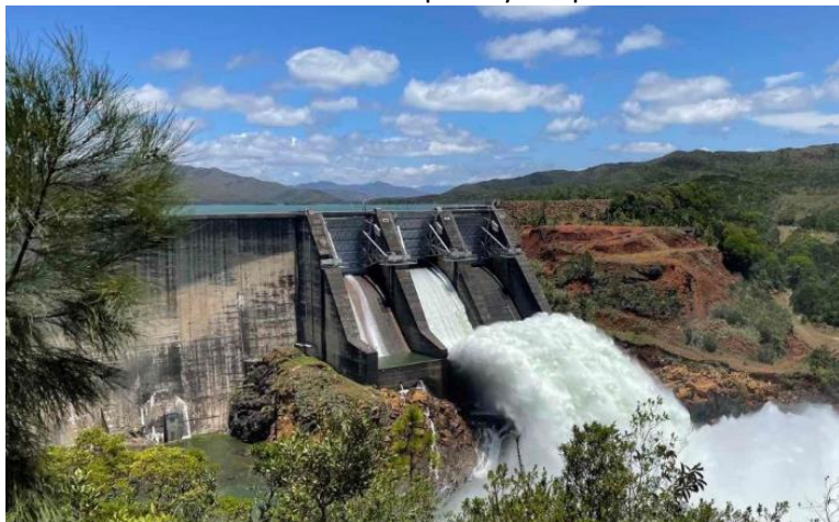
© Photo ENERCAL spillway in operation
