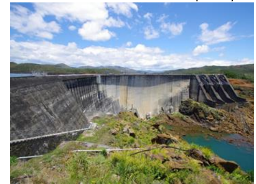
© Photo EDF Arch dam and spillway
