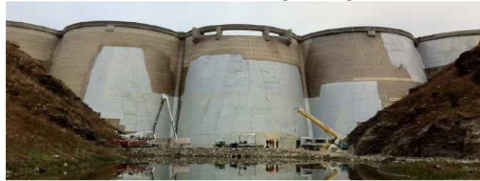
© Photo Somival during sealing works
