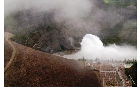
© Photo EDF spillway and bottom outlet exit
