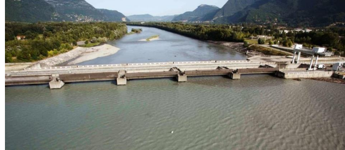
© Photo EDF upstream view
