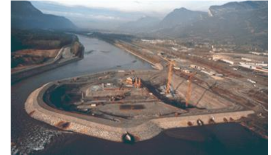
© Photo EDF Cofferdam during construction
