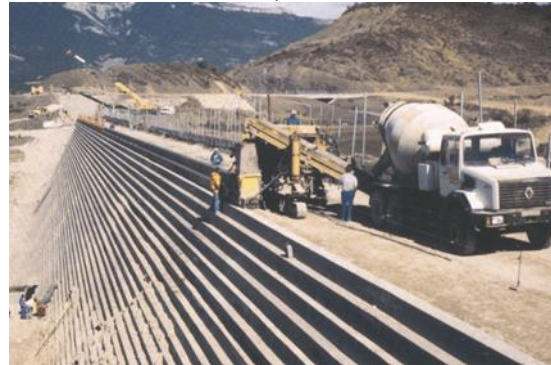
© Photo EDF slipformed concrete
