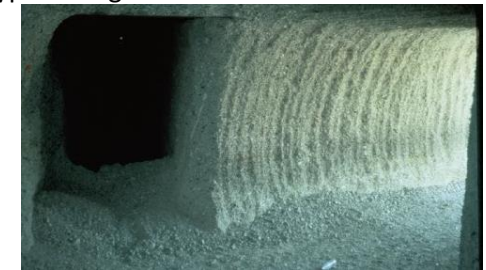
© Photo EDF Gallery excavated with a boom-type boring machine after RCC has hardened
