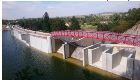
© Photo VNF rehabilitated spillway
