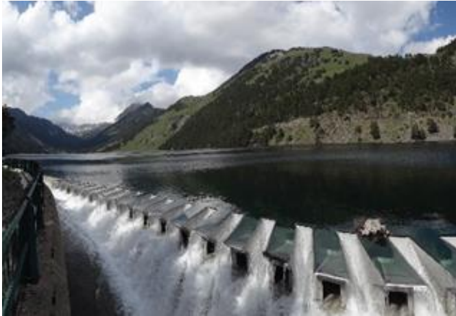
© Photo SHEM Stainless steel PK Weir new spillway
