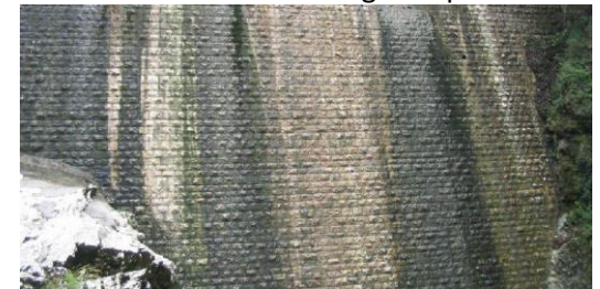
© Photo EDF chute with granit pavement
