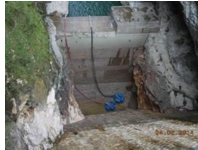
© Photo EDF fosse aval
