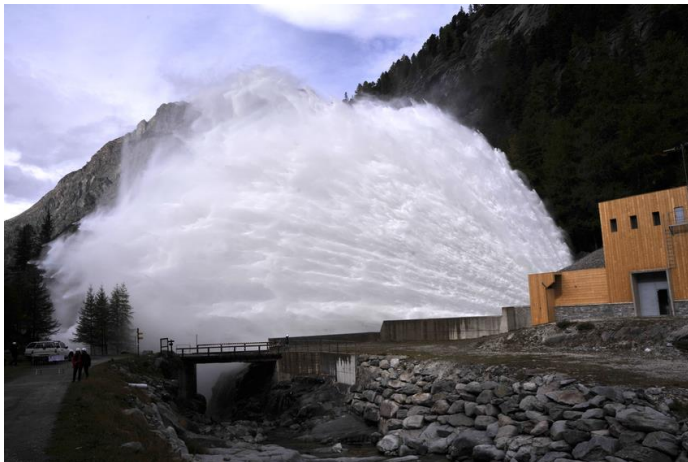
© Photo EDF – Hollow jet bottom outlet valves in operation on french side
