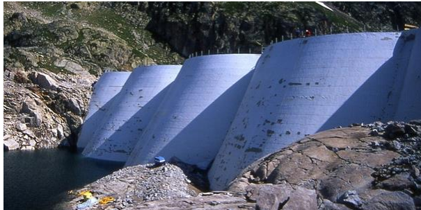
After geomembrane placement © Photo EDF L. Faramond
