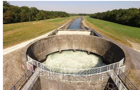
© Photo EPTB SGL stilling basin and return channel to Marne river
