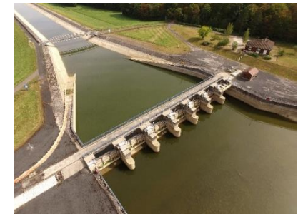
© Photo EPTB SGL gated structure at the end of the entrance Marne channel
