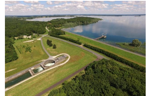
© Photo EPTB SGL gated structure at the end of the entrance Marne channel
