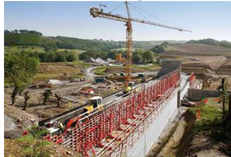
© Photo PERI during construction
