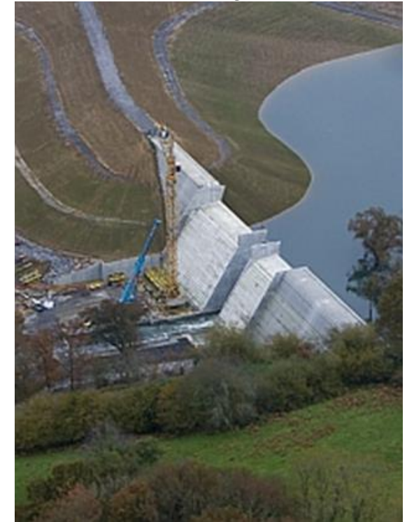
© Photo Vinci during construction
