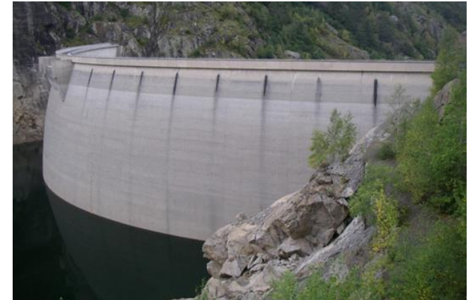
Spillway downstream view © Photo EDF
