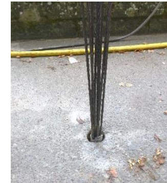
© Photo ISL post tensioned anchors
