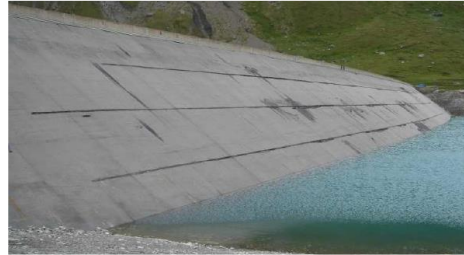
© Photo EDF Bituminous concrete upstream facing
