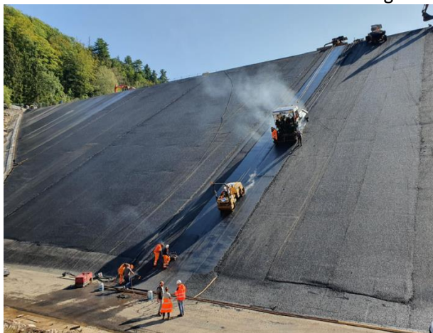
© Photo ISL 2020 New bituminous facing
