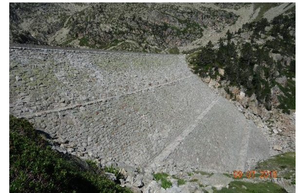
Parement aval © Photo EDF
