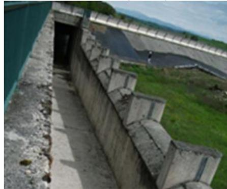
© Photo EDF Spillway chute
