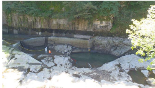
© Photo EDF dissipation basin downstream spillway tunnel
