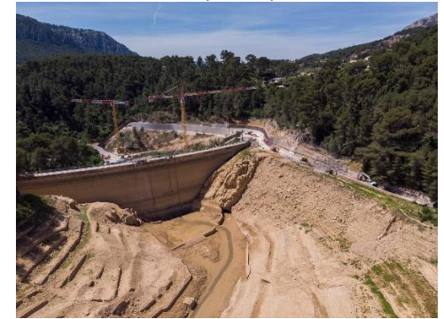
© Photo SCP – Spillway Work (2021)
