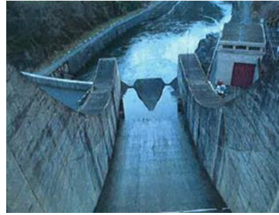
© Photo EDF Right bank spillway chute and ski jump
