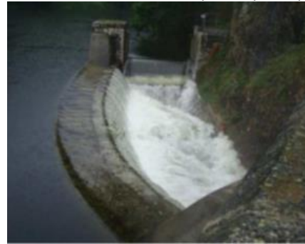
© Photo Roannaise de l'Eau spillway in operation
