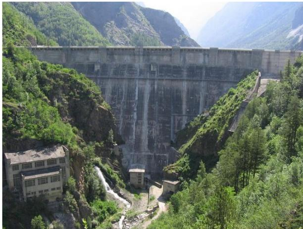
Former surface spillway section concreted in 1994
