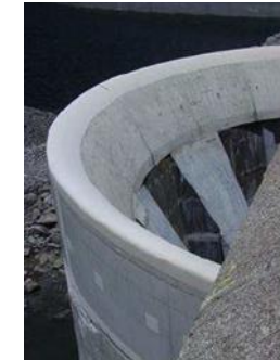
Spillway weir © Photo EDF
