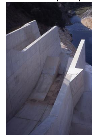
© Photo BETCGB spillway chute
