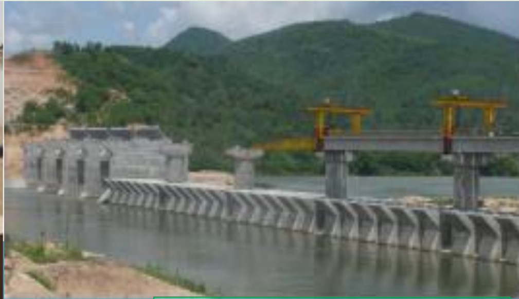
PK Weir of the Dam in Vietnam
