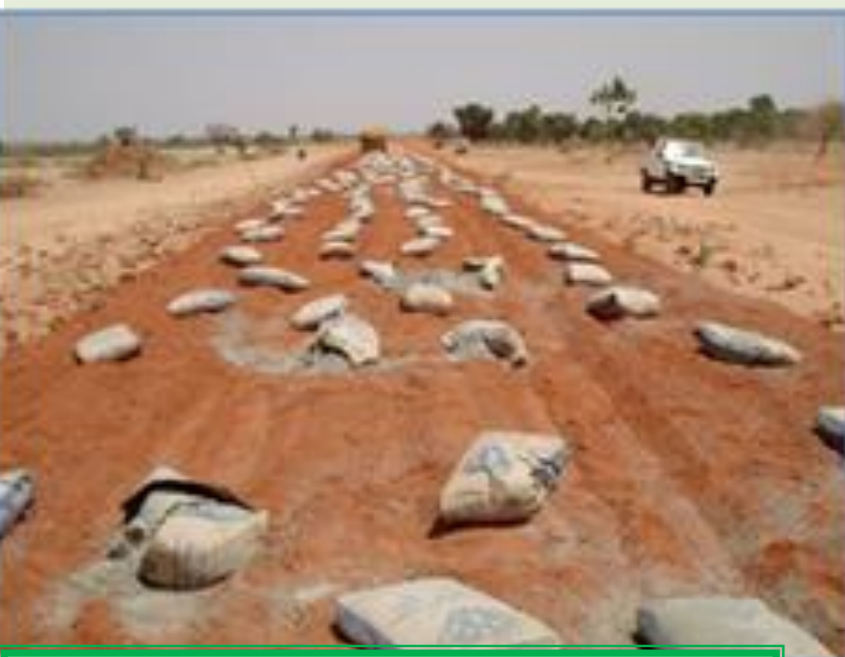
Soil cement placement for Lumbila Dam in Burkina Faso
