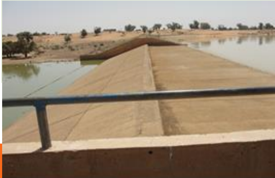
Spillway for the Yakouta Dam in Burkina Faso
