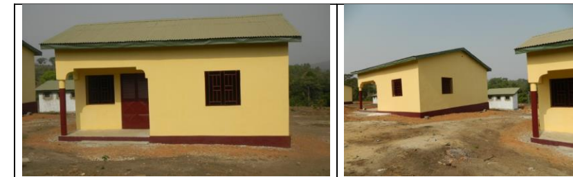
Figure 1: New houses (Silikhoum sites - right bank). TRACTEBEL, 2015
