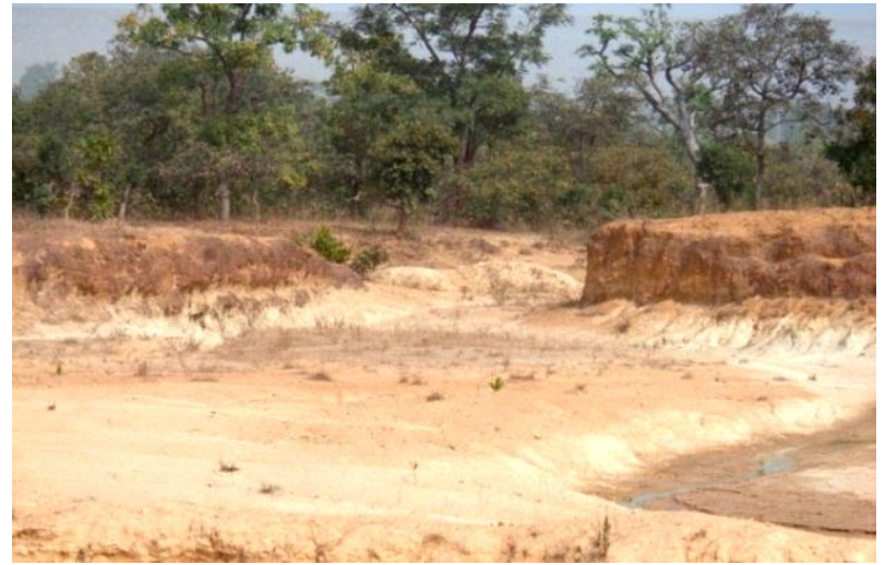
pit created by rock excavation (L) and material borrow area (R) at the Gurara Dam Site
