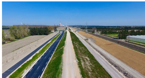
Mainly embankment levees (10 km resisting to overflow)
