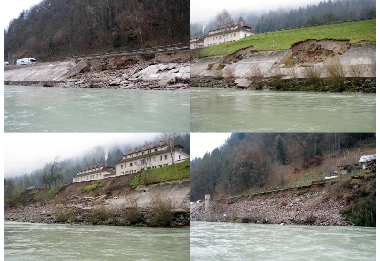
Some examples of damaged banks of reservoirs
