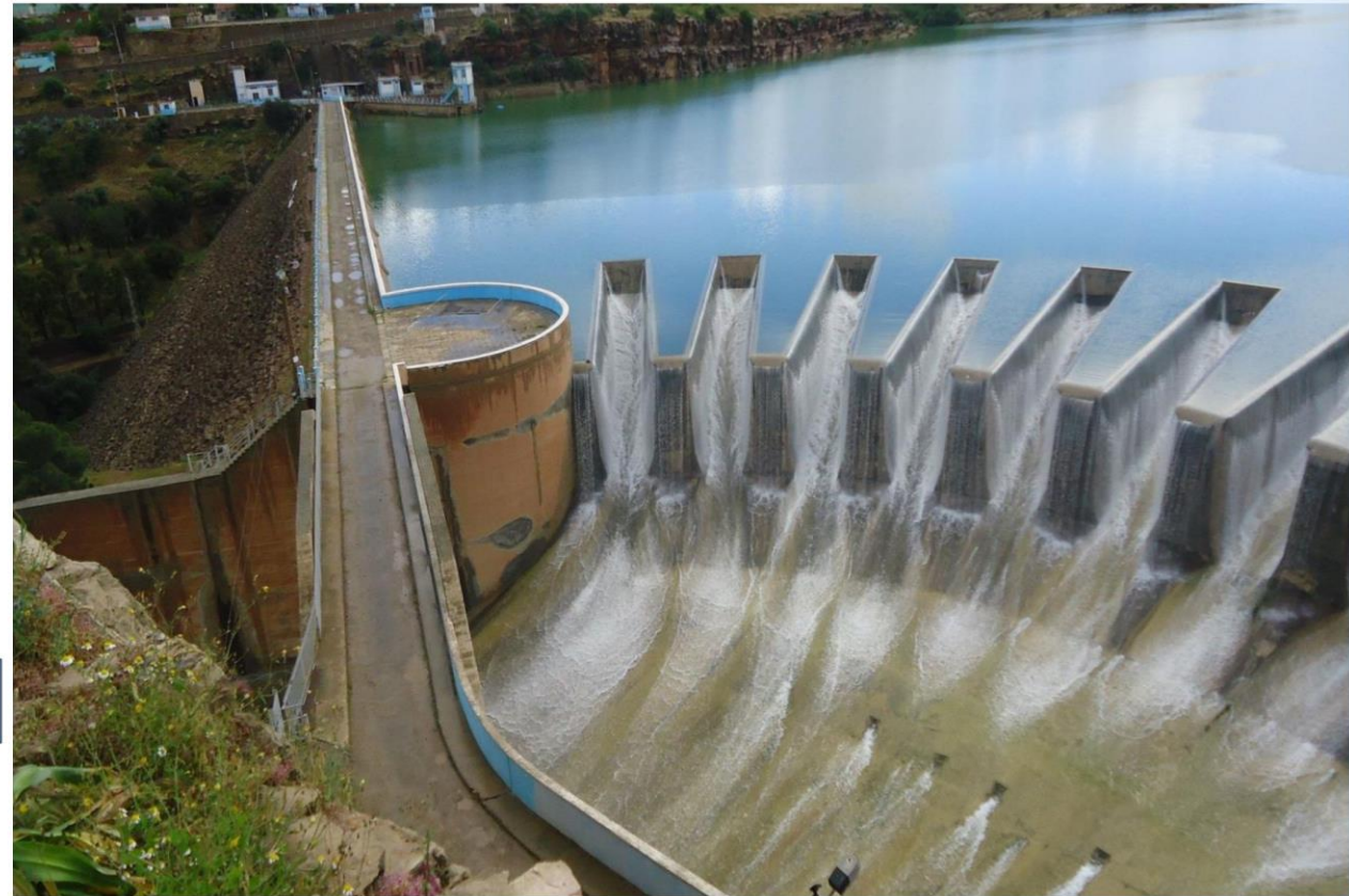
Curved labyrinth weir (after 1960)
