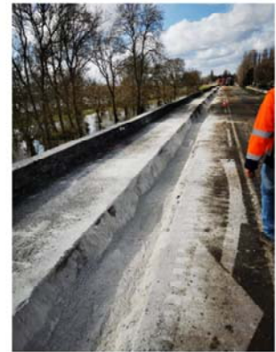
Addition of cement in the pre trench
