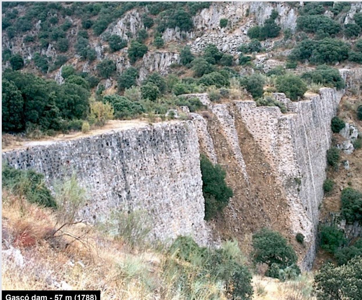
Gascó dam - 57 m (1788)
