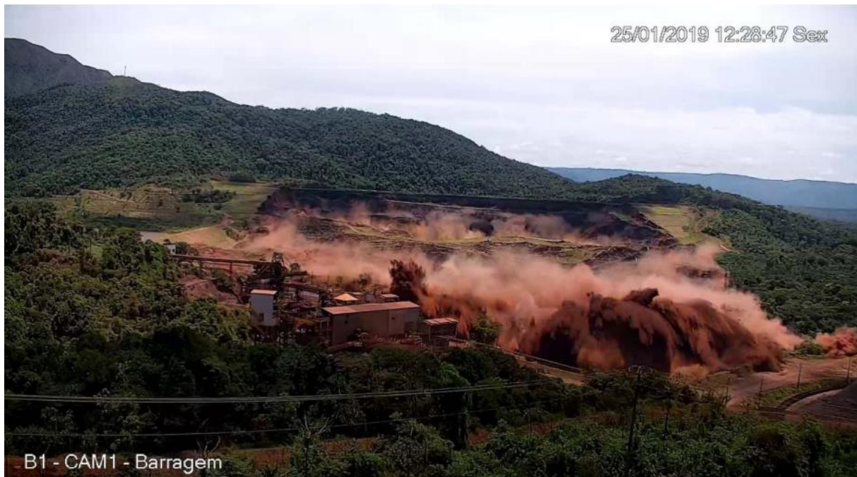
Figure 4: rupture du barrage de Brumadinho
