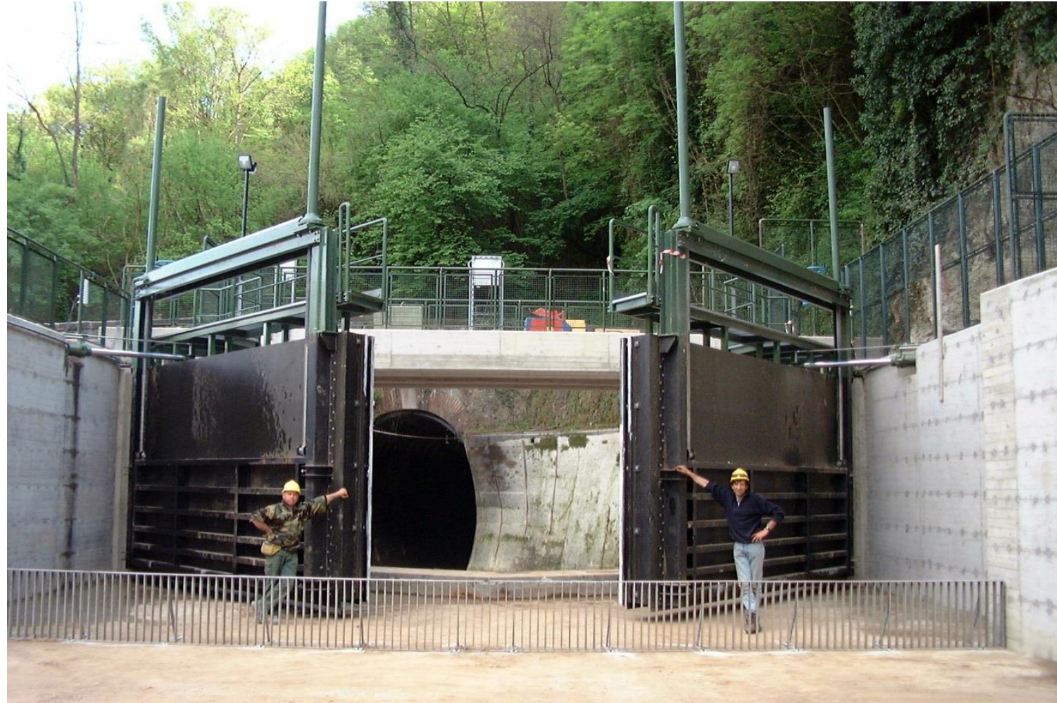
Gate before the tunnel inlet
