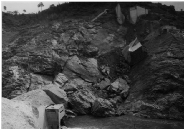
Fig. 7. The 'dihedron', a deep excavation cut inside left valley side at the foot of the dam. The concrete block inside has fallen from the thrust block after the flow (photograph P. Duffaut, May 1960).
