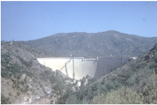
Fig. 1. Downstream view of Malpasset dam close to end of construction: the thrust block appears at right (on the left bank), the spillway weir in the centre (photograph COB, summer 1954).
