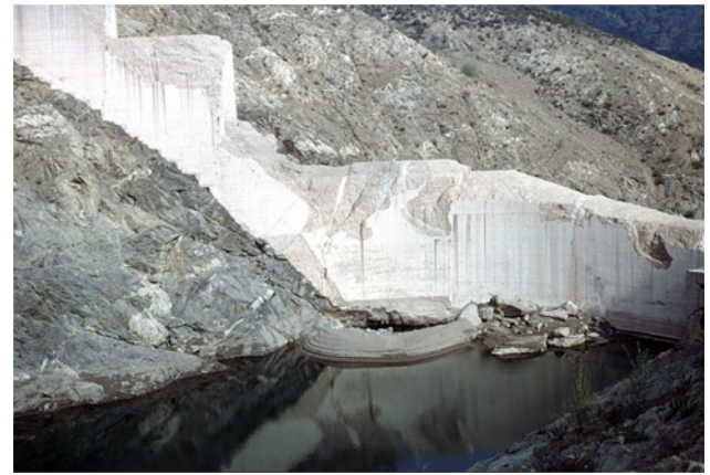
Fig. 12. The debris sill formed underwater by the flow below cantilever FG (photograph P. Duffaut, May 1960).
