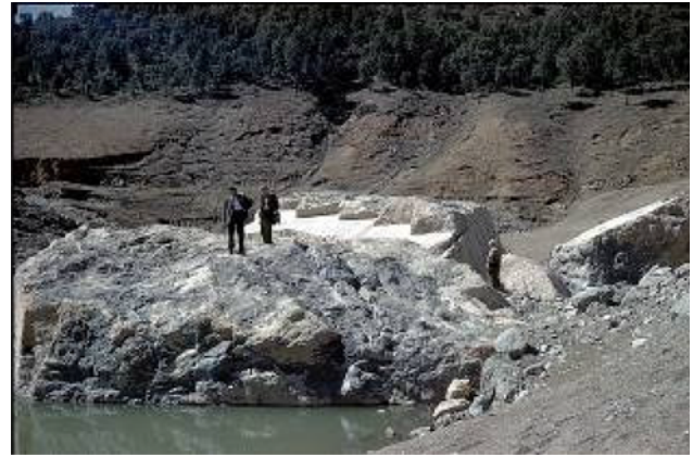
Fig. 9. The two main concrete blocks, 600 m downstream of the dam: on the overturned block, the foundation rock remains adhered to concrete (photograph J. Duffaut, 20 December 1959).
