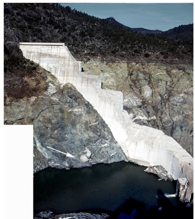
Fig. 6. Remains of the dam on right valley side and valley bottom; the rock appears crisscrossed with white pegmatite dykes; the arrow shows the main fault; the river flow passes through the outlet valve (two assembled photographs, J. Duffaut, 20 December 1959).
