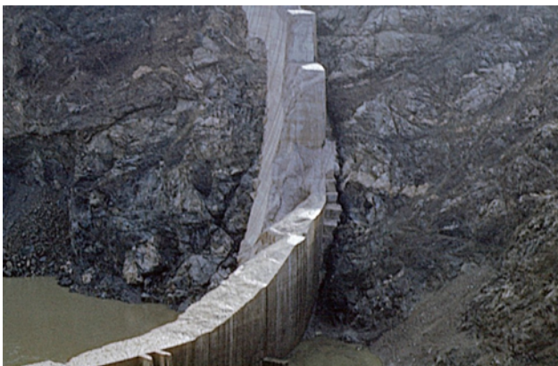
Fig. 8. A conspicuous open crevice separates the dam concrete from the rock mass upstream (photograph J. Duffaut, 20 December 1959).
