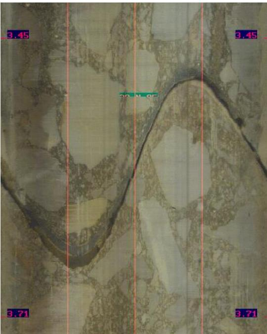
→ The investigations showed internal cracks into the seven cantilevers of the rights banks
